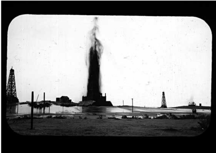
The 1910-1911 Lakeview oil gusher in Bakersfield, California. Oil gushers had a high EROEI as a high-energy fuel was delivered to the surface by natural underground pressure. Early renewables could not match this energy yield for the energy expended. Innovations in the manufacture of renewable generators over a period of decades have now led to significantly higher EROEI for many renewables than for contemporary, more difficult oil extraction.
