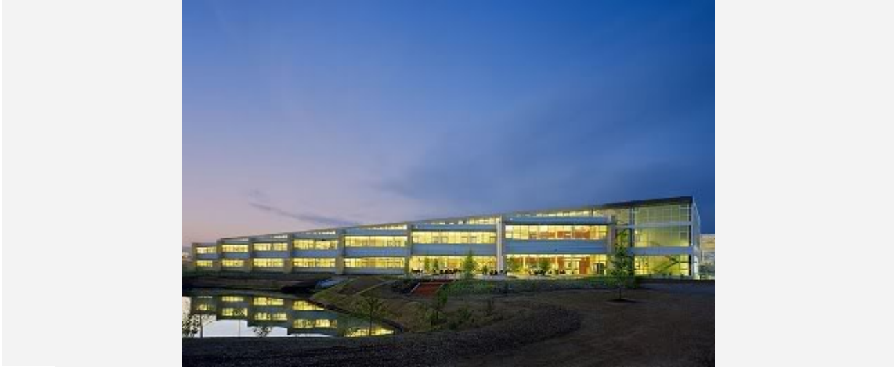
Making a statement about green design, the Alberici construction company of Missouri built their new headquarters as one of the highest scoring LEED Platinum buildings. The architects re-used the shell of a 50 year old manufacturing and office facility, orienting the new facades of the rebuilt structure towards the south to capture more winter sun and optimized natural ventilation flows to increase energy efficiency and improve indoor air quality.
