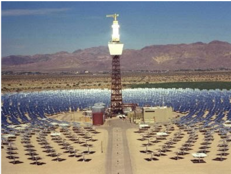
The Solar Two demonstration power plant, built by the US Department of Energy, generated power for seven days and nights continuously using only solar power, which was stored for night time use as heat.
