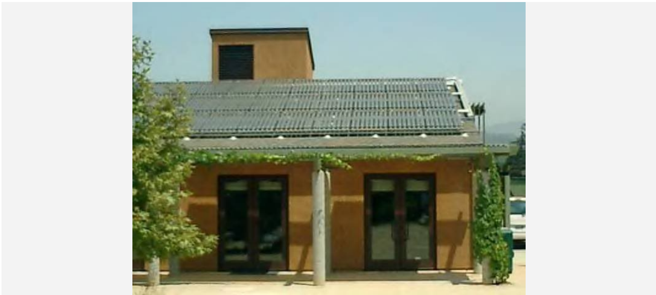
This net zero energy building in Los Angeles, the Audubon Center at Debs Park, has an innovative system of rooftop solar thermal collectors and absorption cooling which use solar heated water to both heat and cool the well-insulated interior space (also a LEED Platinum building).
